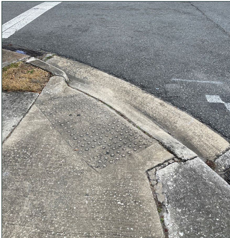
Existing Tactile Pad at St. Augustine Road near Auburn Road Source: Project Team
